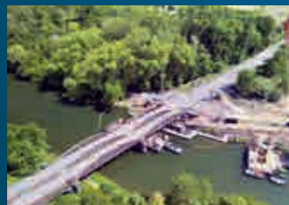
UK: Nuneham rail viaduct restoration, Network Rail.
