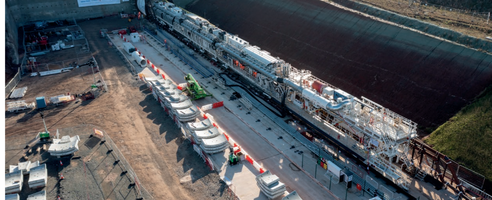
HS2 Main Civil Engineering Works
