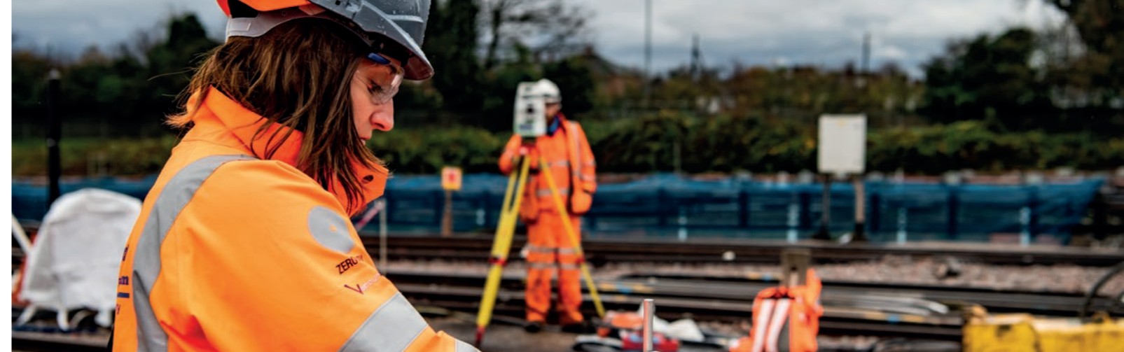
London Underground Track Renewals
