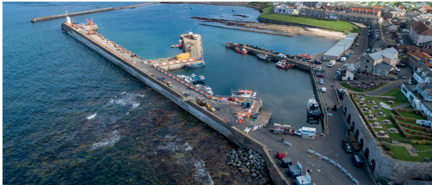
Seahouses Main Pier Refurbishments
