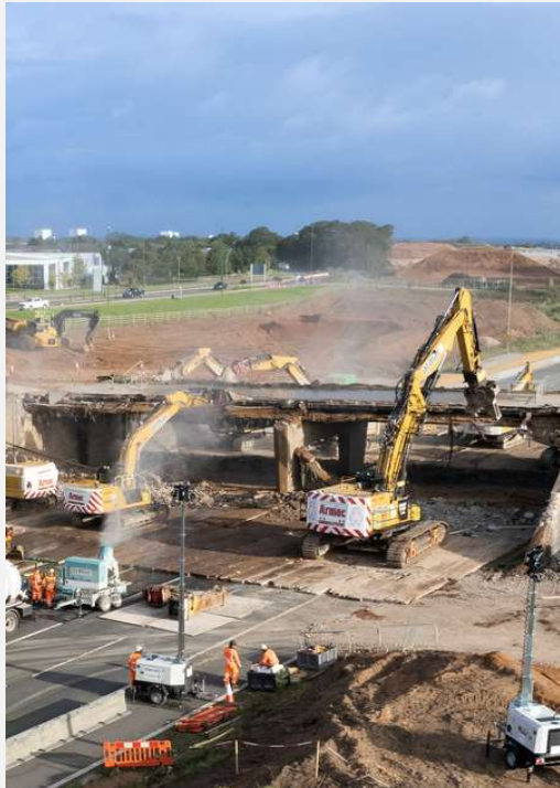
M42 bridge demolition
