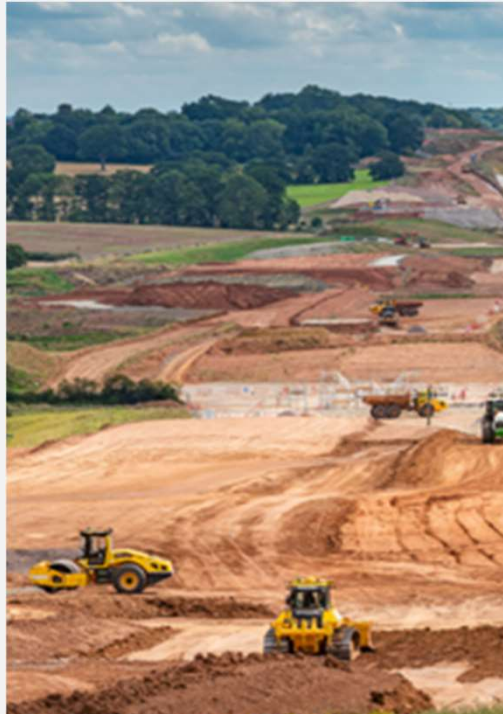
Cubbington cutting earthworks
