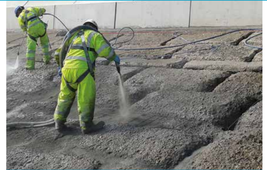
Spray concrete repairs to revetments at Grimsby
