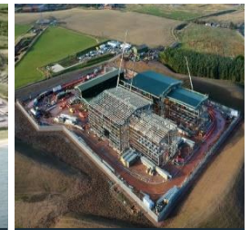
Offshore wind connection and base construction
