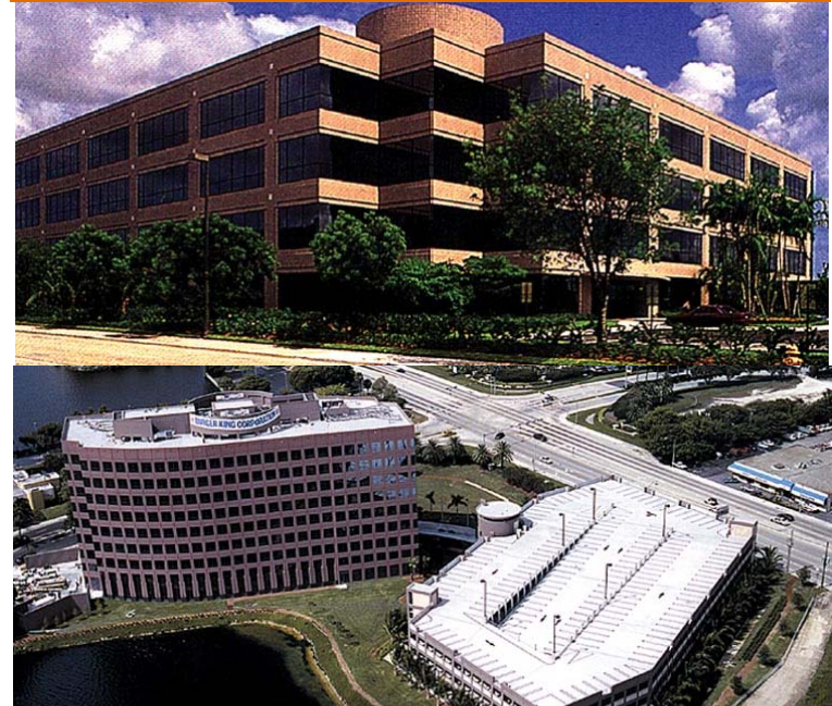
8 Waterford Office Projects
