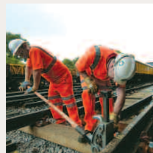
Above: Track renewals on the London Underground – Balfour Beatty Rail Projects.
