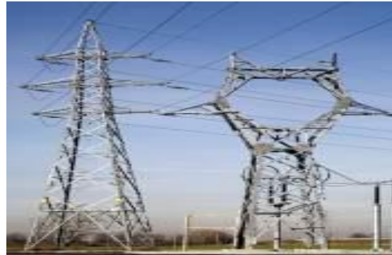
Overhead Line Upgrade (USA)
