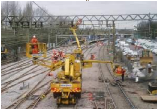
Track Renewal RT24
