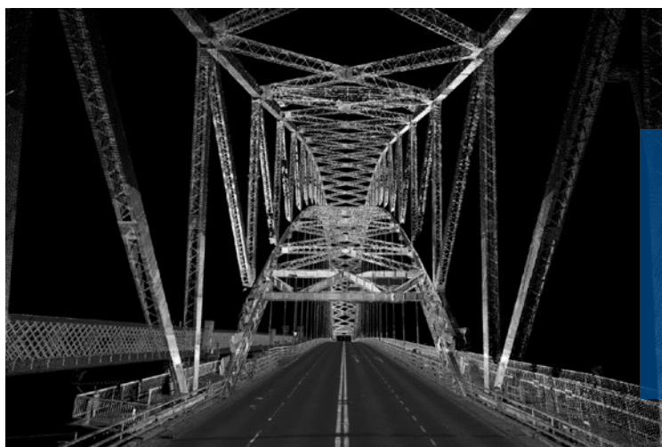
Silver Jubilee Bridge, Halton, UK Balfour Beatty has developed its own in-house specialist scanning teams that use the latest software to capture existing historic structures for future maintenance works.
