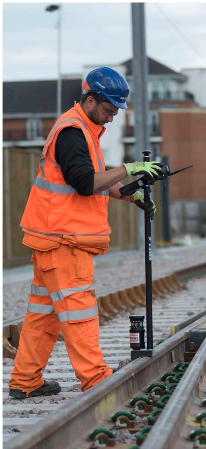
Crossrail Abbey Wood Station
